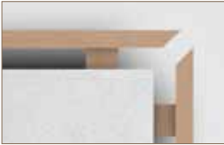
open miter joint
