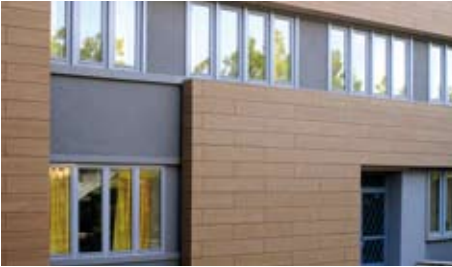
school building | Athens
