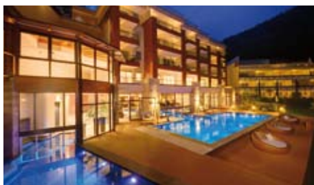
outdoor hotel facility | Meran
