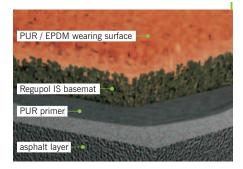
The professional surface featuring a very comfortable level of force reduction similar to the traditional Regupol AG system. It is a 'sandwichtype' surface structure whereby the 'insitu' basemat is installed on site by mixing the rubber granules and the PUR binder before
