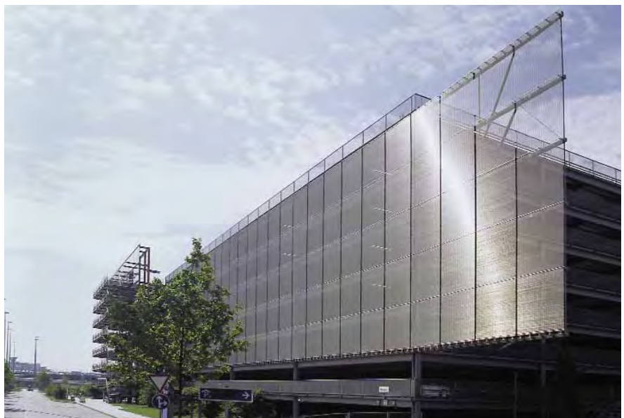
Facade Design with Woven Wire Cloth Elements made from Stainless-Steel, Car Park P3, Airport Cologne/Bonn
