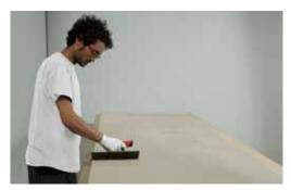
Apply the adhesive with the back-buttering method in full bed, first on the slab back side and then on the substrate, caring to cover corners and edges, too, and avoid air gaps between substrate and slab. Apply the adhesive gradually only on the surface involved in the application of a slab, to avoid surface film that could jeopardize bonding.
