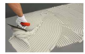
The choice of the squeegee to be used depends on the finishing and flatness of the substrate and is directly proportional to the slab dimensions. Generally, for a slab **1000x1000 mm**, it is recommended to use a squeegee with 6-mm sloped teeth for the substrate and a squeegee with 3-mm sloped teeth for the slab back side.
