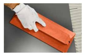
Beat on the surface using a rubber coated squeegee caring to eliminate gaps and air bubbles. Always check the perfect adhesion of corners and edges. Do not walk on the floor during and after the application, respecting the trampling time indicated by the adhesive manufacturer.
