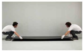
Overlap several slabs horizontally, making sure the surfaces are clean and the supporting plane is perfectly flat.
