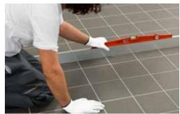
Check for the flatness of the screed or of the existing floor Flatness differences can be smoothed by self-levelling products.
