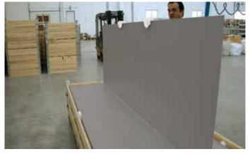
Position the package close to the surface to be coated. Lift the slab from the long side till positioning it vertically.
