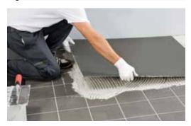
Lay the slab carefully on the long side and, keeping it slightly sloped, lower and apply it and make it adhere on the substrate.
