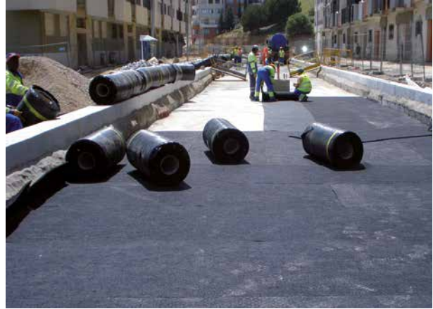
The picture on the left shows the laying of Regupol® SB 16/100 prof , a tried and tested elastic intermediate layer for light mass-spring systems, in Almada, Portugal.
