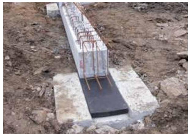
Strip decoupling of a building foundation with Regupol®/ Regufoam® vibration damping material: 1 natural surface • 2 impedance plate • 3 Regupol®/ Regufoam® vibration isolation • 4 foundation plate • 5 basement wall • 6 floor slab
