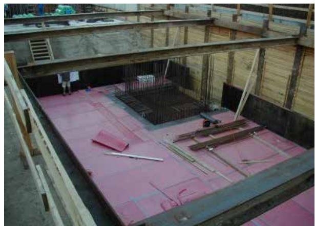
Full-surface decoupling of a building foundation with Regupol®/Regufoam® vibration damping material: 1 natural surface • 2 impedance plate • 3 Regupol®/Regufoam® vibration isolation • 4 foundation plate • 5 basement wall • 6 floor slab
